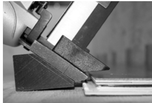
Fig. 9 Nail gun lifted over the locking element
