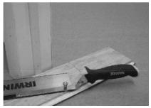
handsaw or use a power jamb saw set at the correct height. Remove all moldings and wall-base, and undercut all door casings.
