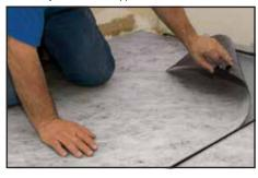
2.10 For a proper bond between *Mapesonic 2* and the tacky floor, roll a 75- to 100-lb. (34,0- to 45,4-kg) roller over the installed membrane. For smaller pieces of membrane, use a wood float or steel trowel to apply pressure.
