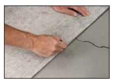
1.4 Set aside precut sections (or entire rolls) of *Mapesonic 2*. Continue with installation instructions at Step 2.3.
