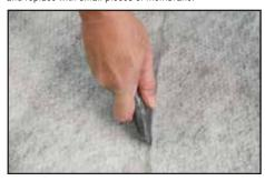
2.12 Layout lines for tile, vinyl or wood can be easily applied and viewed on the light-colored membrane.
