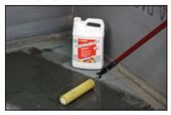
2.8 Apply the membrane (at the previously marked starting point) to the tacky substrate.
