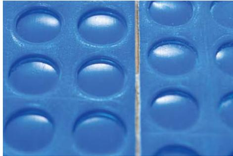
9. Lift the membrane occasionally to verify coverage. Proper installation results in full contact between the fleece layer backing and the mortar.
