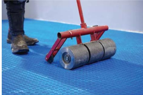
8. While laying the rolls of the membrane, it is recommended to leave a 3- to 5-mm gap between the sheets. To ensure a flat surface, do not overlap edges or ends from one roll onto another. Leave about 1/4" (6 mm) between the membrane and the edge of walls, columns, etc., for movement.
