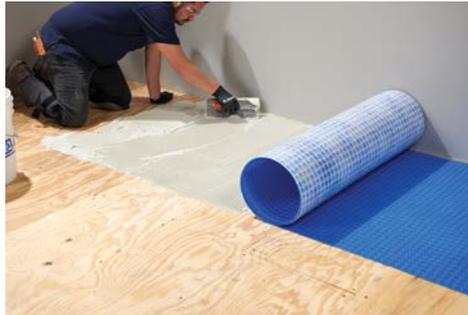
6. Spread only as much mortar as can be covered with *Mapeguard UM 35* [NA] before the mortar skins over. Open times vary with jobsite conditions and mortar choice.
