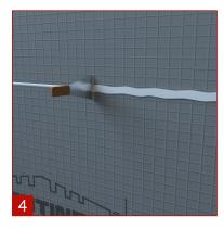
4. Use a putty knife to spread polyurethane adhesive flat over all joints.
