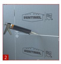
2. Apply polyure than eadhesive on the joints which are between the boards.
