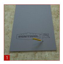
1. Cutting the SENTINEL CEMENT FOAM BOARD into suitable size.
