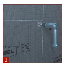
3. Fasten the board to a stud using Sentinel Stainless Steel Washers and Screws .
