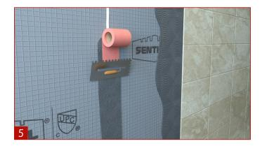
5. To help avoid leaks, cover all joints with Sentinel Waterproofing Seam Tape.
