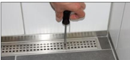
SQUARE grate assembly with locking mechanism
