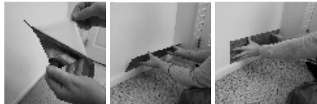
3. Once the first panel is placed, continue installing panels in the same horizontal row, completing one row before moving vertically to the next row.
